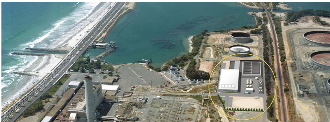
Figure 1: The Carlsbad Desalination Plant being constructed on industrially zoned land adjacent to the Encina Power Station in Carlsbad, CA. Photo: © 2016 Carlsbad Desalination Project, http://carlsbaddesal.com .
