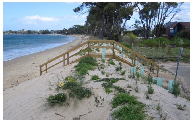
Figure 1: Filling in low points, new stepped access and revegetation — Lauderdale. Source: © Clarence City Council 2012.
