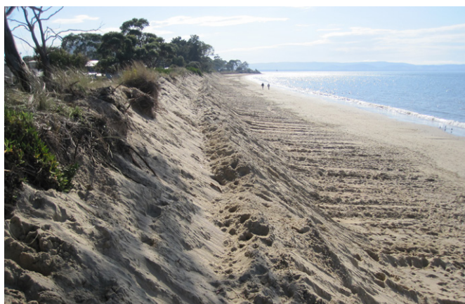
Figure 2: Dune nourishment using beach scraping — Lauderdale Beach Tasmania. Source: © Clarence City Council, 2011.
