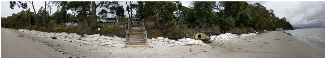
Figure 6: Initial stages of the sandbagging project have been undertaken by Council to protect Coningham Beach from coastal erosion. Photo: © Kingborough Council, 2016.
