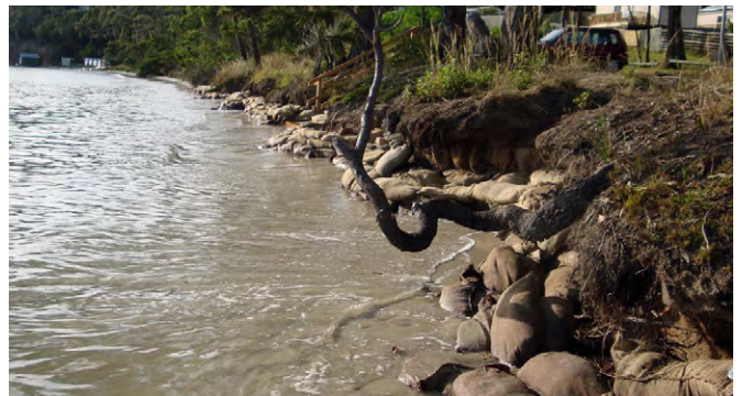
Figure 5: Coningham Beach experienced a 'King' high tide event on the 24 th of January 2011. Sandbags and replanting of coastal vegetation were used to protect the shoreline against erosion. Photo: © P. Donaldson, 2011.
