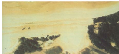
Sheltering Palms, 28 th August, 1977 All trace of the village has been removed. An artificial dune constructed by pushing sand from the washovers into a pile along the front of the beach is complete. This is intended to serve as a temporary buffer to prevent breakout of the river to the ocean.
