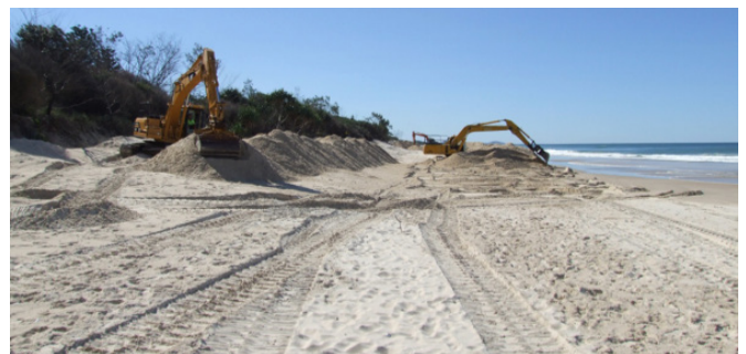
Figure 3: Machinery at work during beach scraping. Source: © Byron Shire Council 2013.
