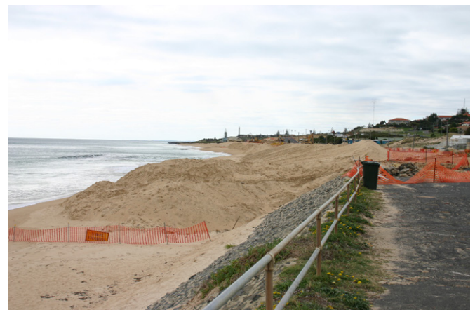
Figure 2: Works in Back Beach, Bunbury. Photo: © Garry Middle.
