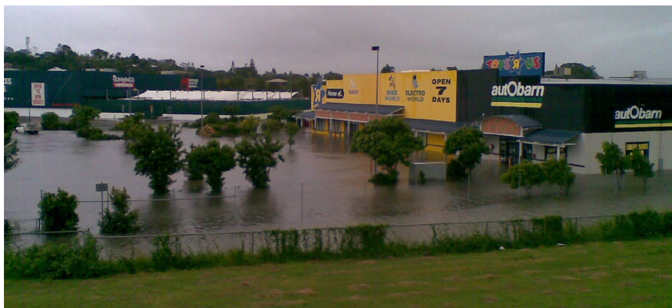
Figure 1: Major flooding in a shopping centre at Mackay. Photo: © Robyn Birkett.
