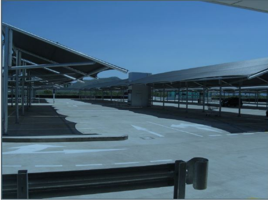
Shade structures added to the carpark for customer comfort. Source: Johnson, 2013
