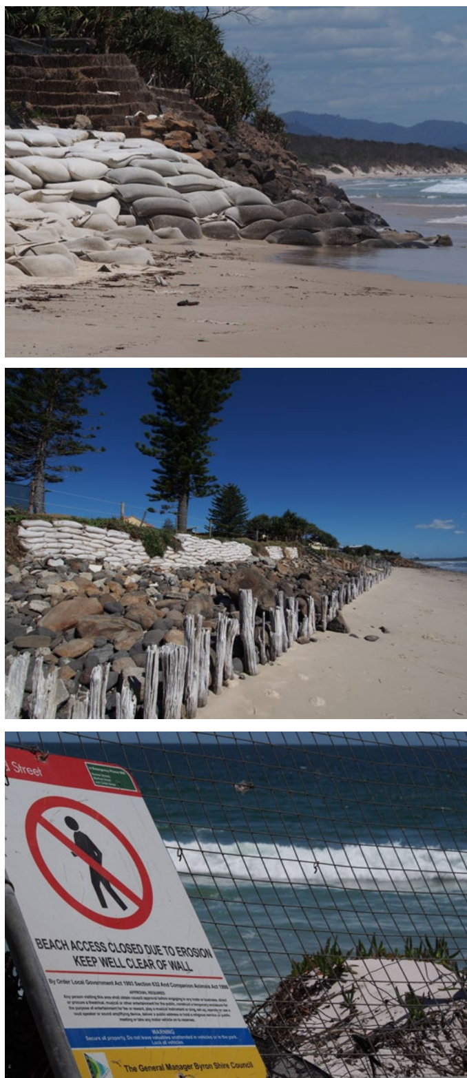
Figure 1: Beach profile modification through seawall construction and sand renourishment activities. Photographs: © Dana Thomsen.
