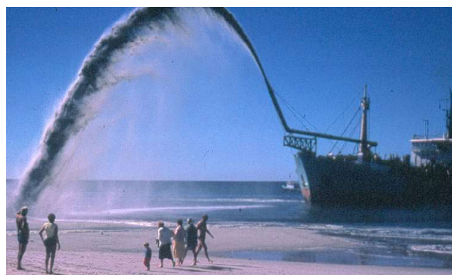
Figure 18: Sand nourishment pump in action, Woorim, Bribie Island. Source: © The State of Queensland (Department of Environment and Heritage Protection).
