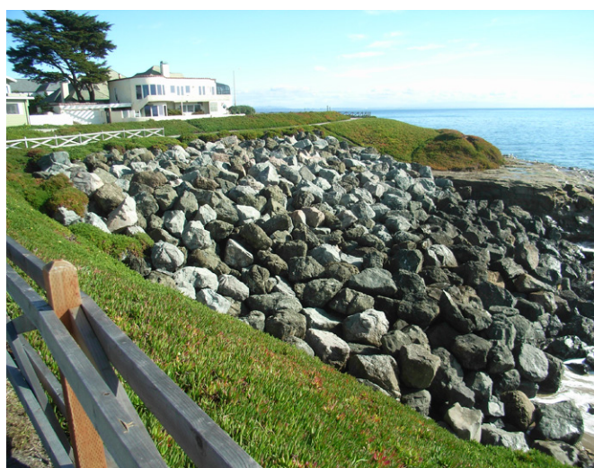
Figure 16: Random-placed rock armour protection – Half Moon Bay, CA, USA. Photo: © 2007 Tony Webb.
