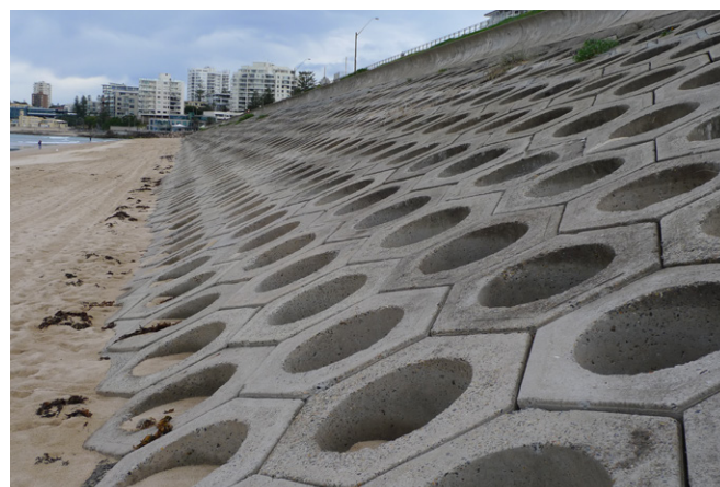
Figure 17: Pattern-placed concrete armour units (Seabees) – Cronulla, NSW. Photo: © 2005 Tony Webb.
